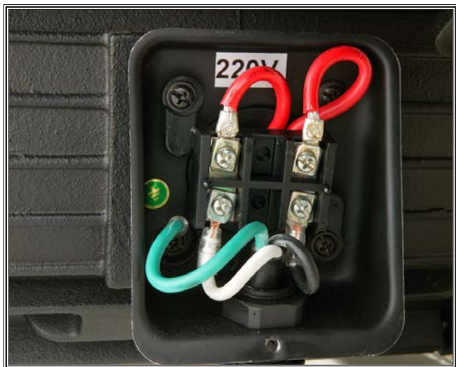
Figure 79. Motor wiring.
